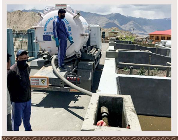
Figure 15: Discharging of faecal sludge at Leh FSTP
